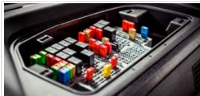
In-cab electrical panel
